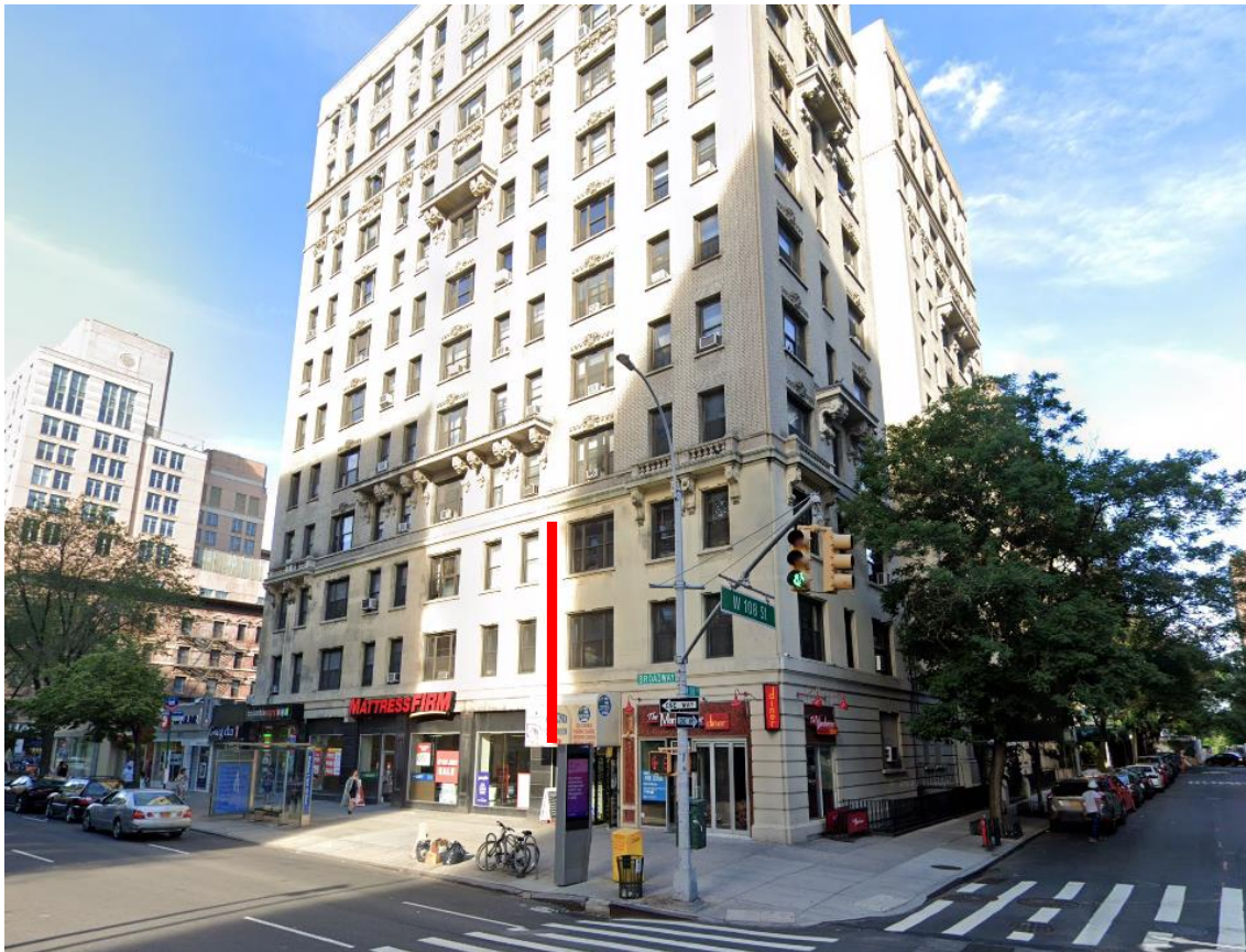
Image 3 - The proposed Link5G tower (to replace LinkNYC kiosk at lower center) will rise nearly to the carved and colonnaded balcony on The Manchester (see red arrow) which was completed in 1910 just a few years after The Manhasset and is directly across Broadway (Source: Google Maps. July, 2019 – to show building without temporary scaffolding.)
