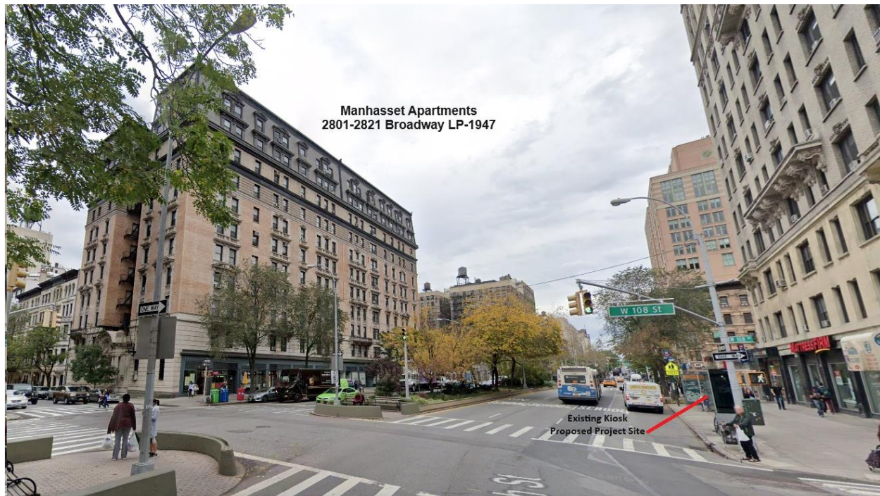
Image 1 – Looking north on Broadway from West 108th St towards Manhasset Apartments which occupy entire west block front. The red arrow shows the existing LinkNYC kiosk, which is the proposed Link5G site location. Tower height will reach to just below fourth floor windows of the 113-year-old Manchester Condominium which is the “backdrop” to the right. (Source: Google Maps October 2017.)
