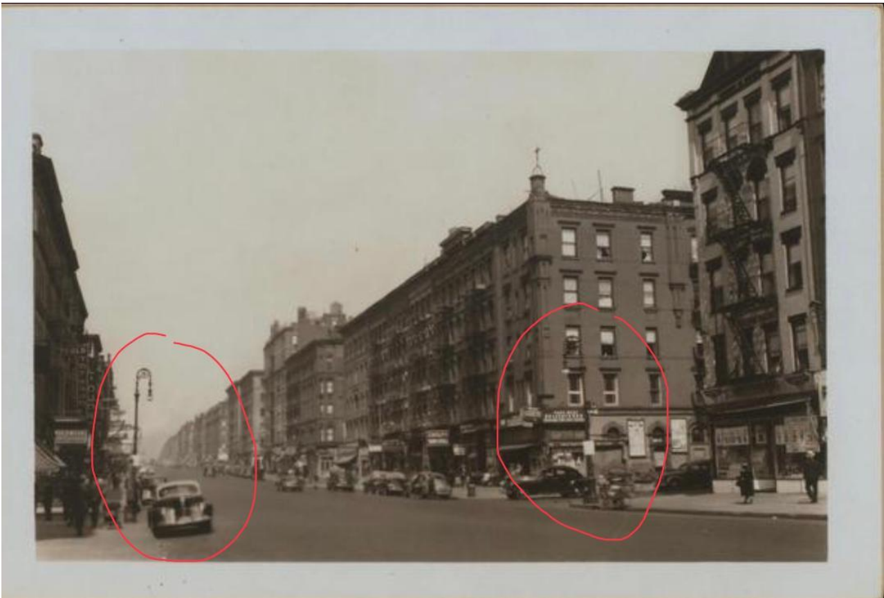
Image 6 – Looking north up Columbus Avenue at W. 83rd Street circa mid-1940s. Two Bishop's Crook poles on opposite sides of intersection are highlighted with red circles. (Source: NYPL Archives)
