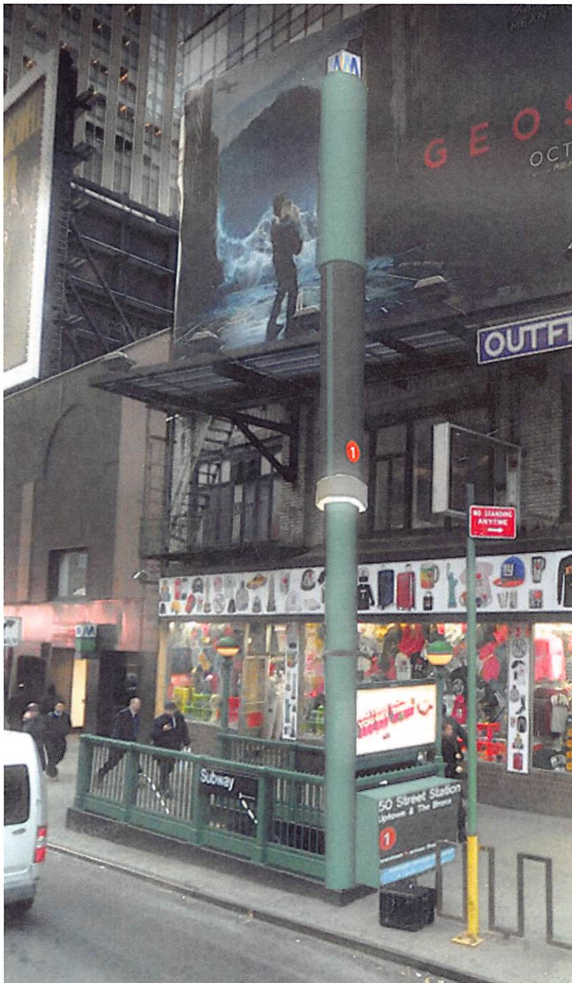
Figure 8-18: MTA Infrastructure Design with Sign Cabinet
