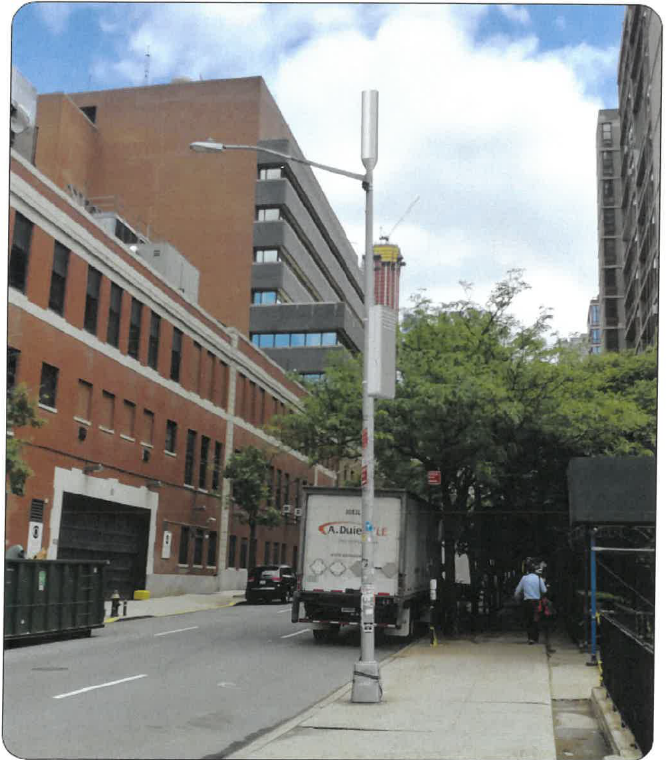
Figure 3 – Photosimulation of resilient shroud with multi-technology antenna solution.
