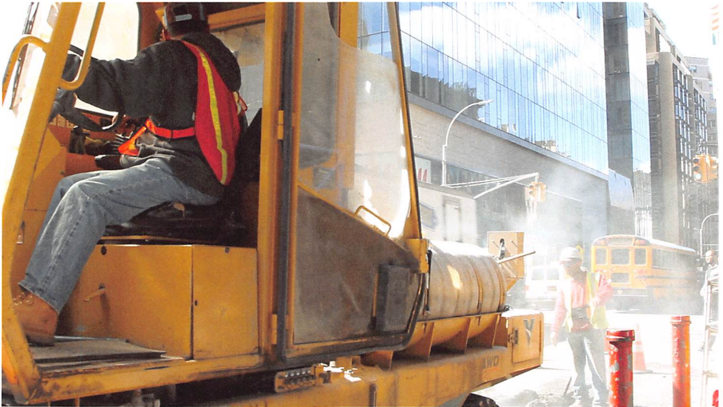
Image 14 - Transit Wireless Experience with Trenching
