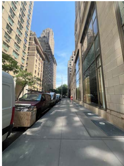
6. View E from Project Site beyond which is Central Park West Historic District (90NR00905) and Upper West Side/Central Park West Historic District (06101.023389)
