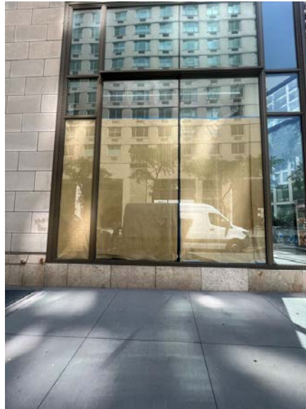
7. View S from Project Site
