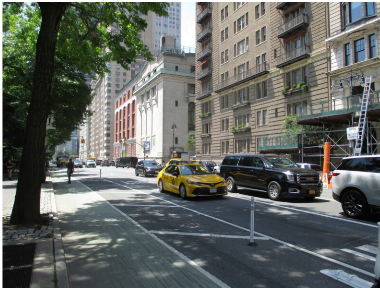
22. Looking southwest at the Upper West Side/Central Park West Historic District, and Central Park West Historic District 500 feet from the Project Site
