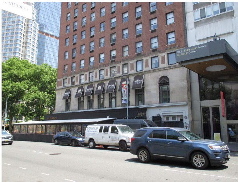
28. Looking northeast towards the Project Site (not visible) from Lincoln Center HD and 500 foot APE-VE Radius
