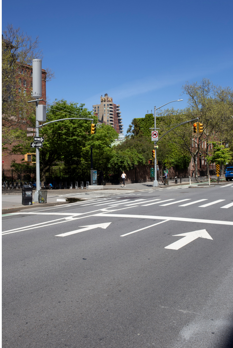
M2 Traffic Signal Pole
